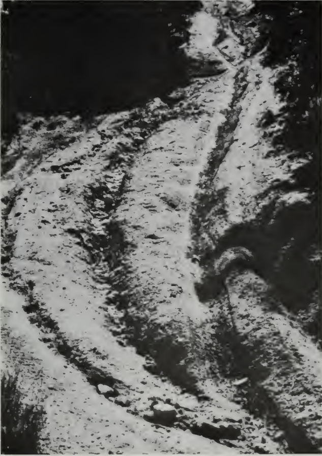
Fig. 3. Trail 15E, designated open with water bars or open top drains and debris basins as mitigations.
