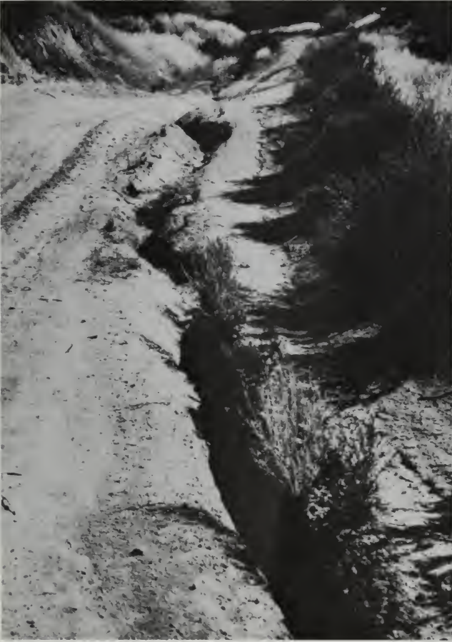
Fig. 5. Trail 150A, designated open with water bars, gully plugs, and fill as mitigations.
